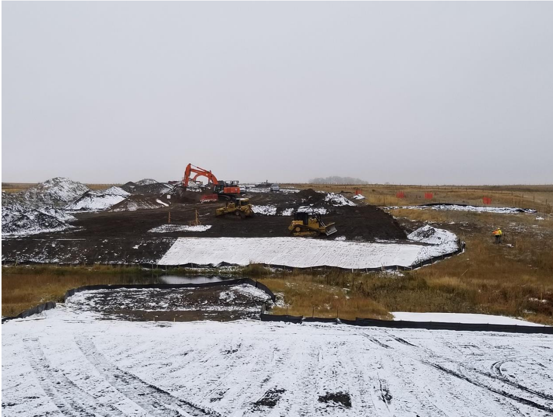
Clean up crew installing diversion berms and moving soils.
