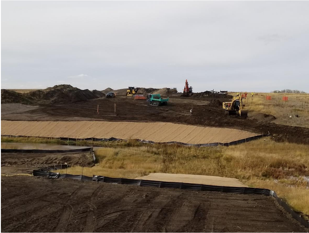
Installation of coco matting on the slope.
