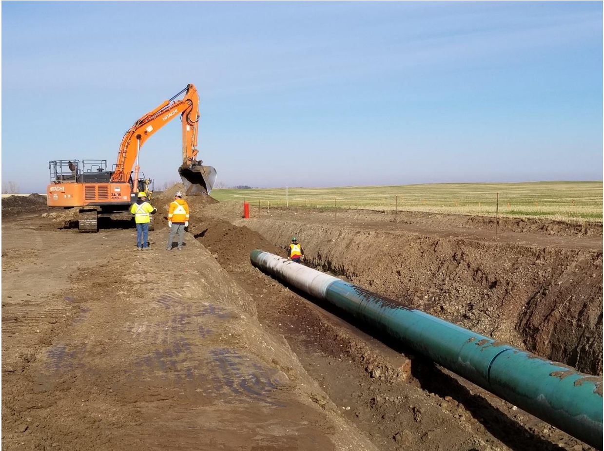
Backfilling a test point.
