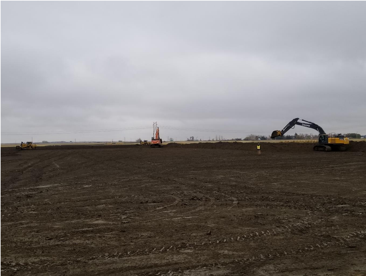
Placing topsoil back over an old equipment laydown yard.
